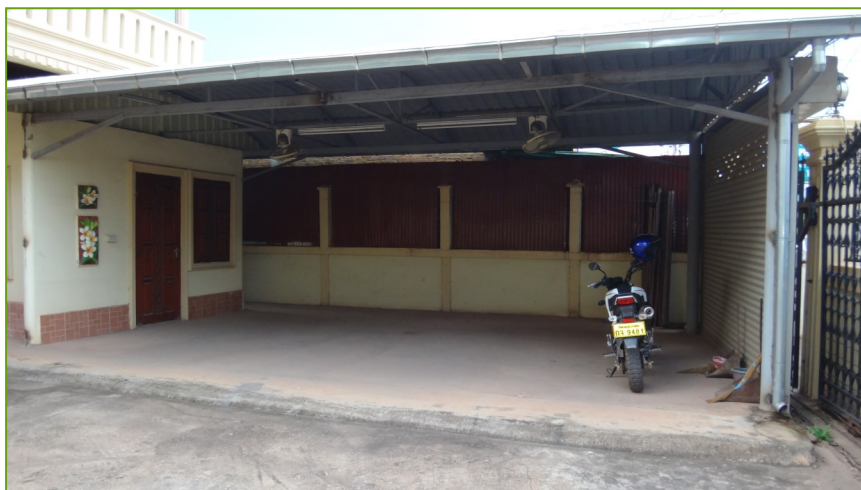
Space that can be converted into a restaurant
