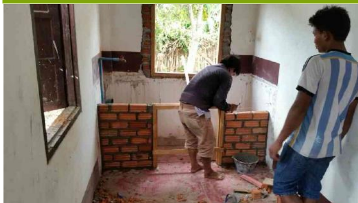
Work on external wall—making air vent and window for kitchen
