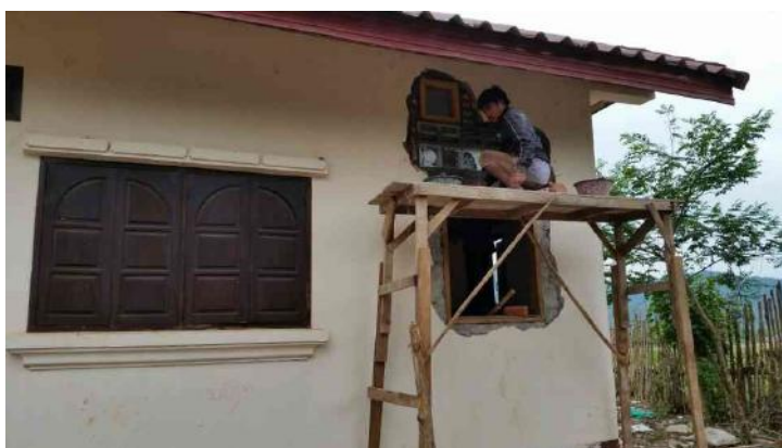
Work on external wall—making air vent and window for kitchen
